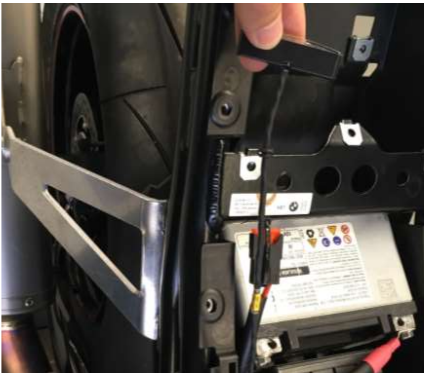
Image 20: Rainlight, main fuse, and battery.
